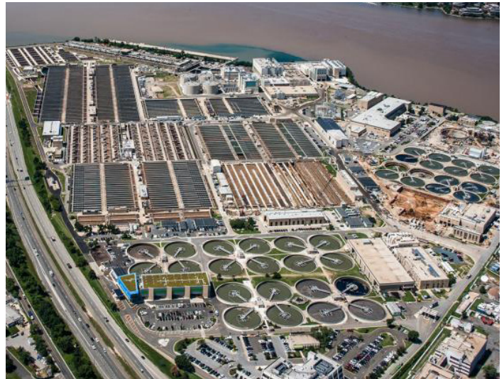
DC Water's Blue Plains Advanced Wastewater Treatment Plant
