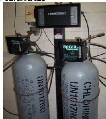
(U) 150-pound chlorine cylinders at a water treatment facility
