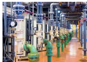
Water and wastewater systems
