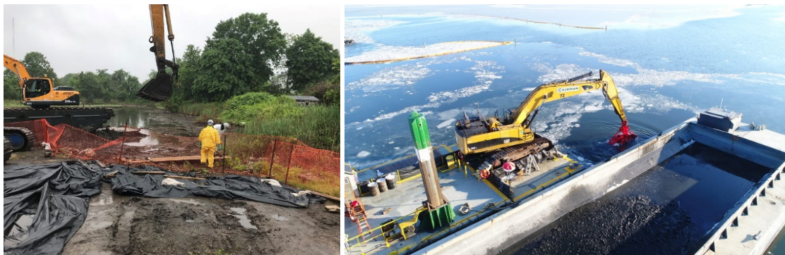
Figure 70: Remediation of polychlorinated biphenyl (PCB)-contaminated soils and sediments in New Bedford Harbor
