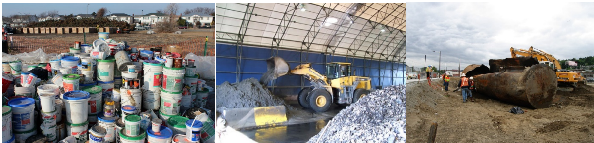
Figure 71: Storage options for hazardous household waste (left), contaminated sediments (middle), and volatile organic compounds (storage tank, right)
