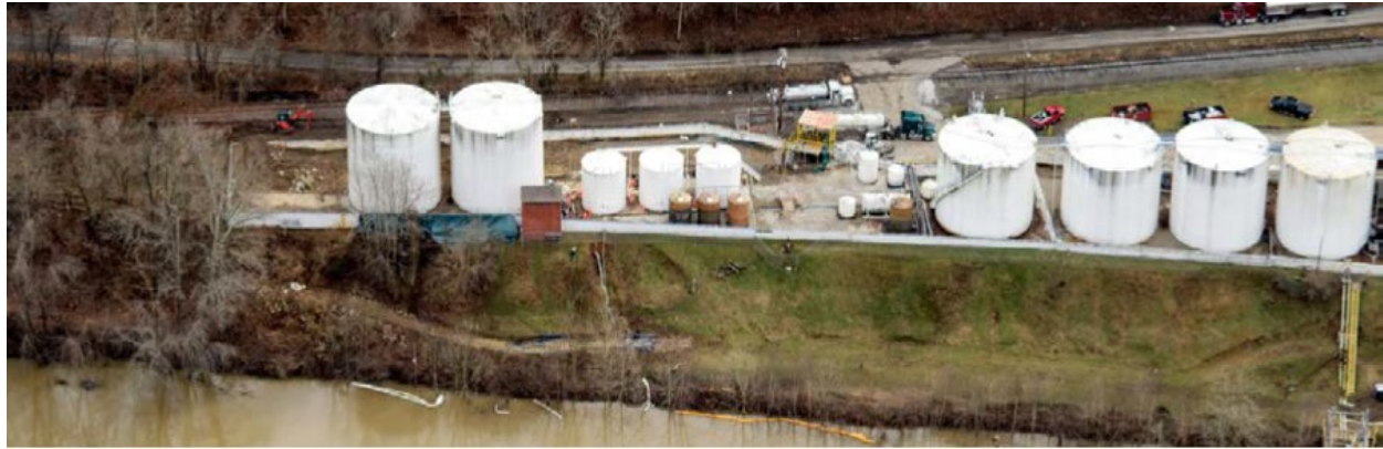
Figure 6: Chemical storage tanks alongside the Elk River near Charleston, West Virginia
