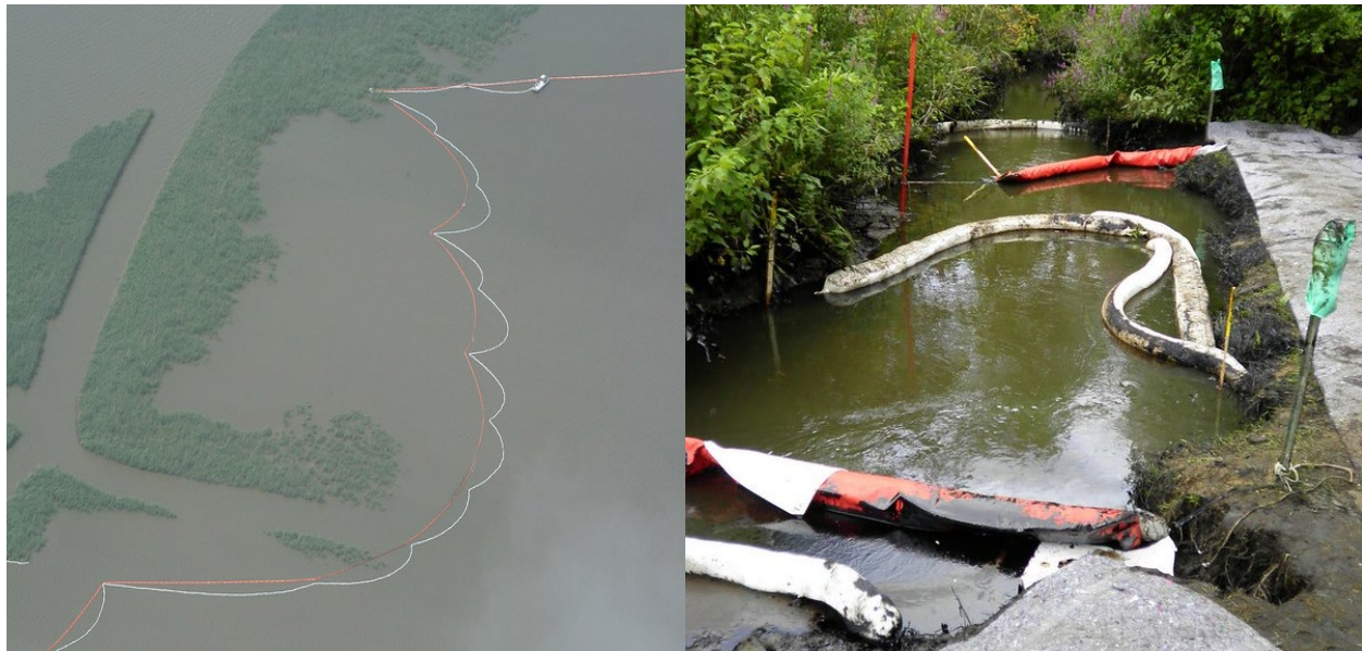
Figure 52: Containment booms on large and small bodies of water
