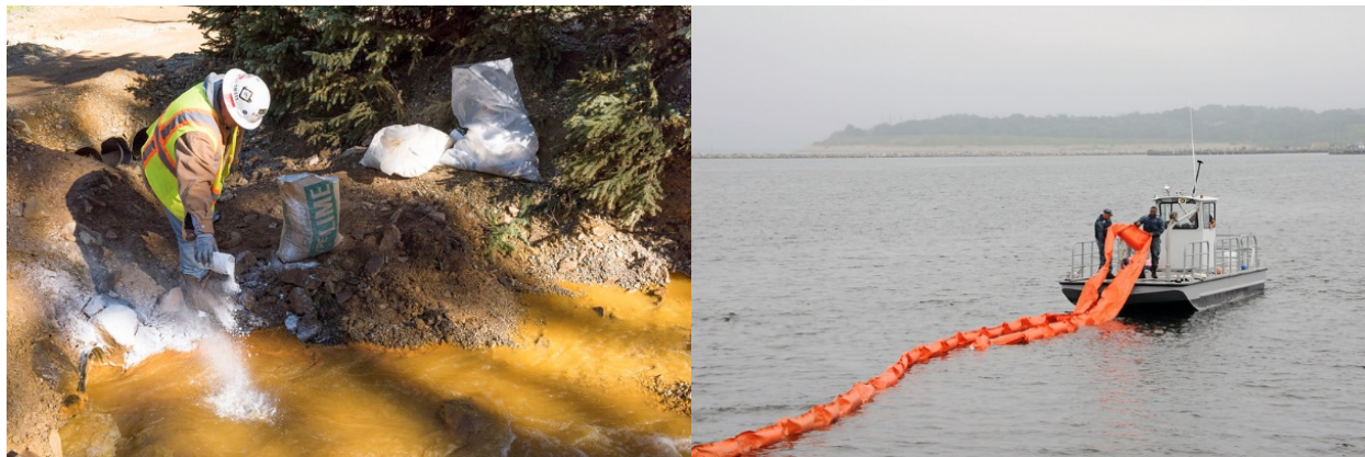
Figure 49: Containment control mechanisms: neutralizing mining wastewater (left) and moving an oil containment boom (right)
