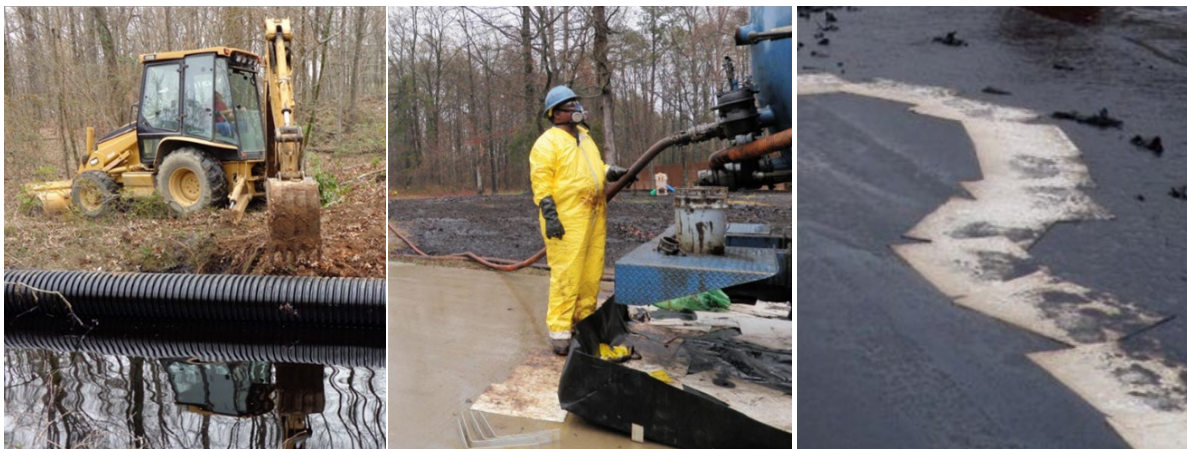
Figure 50: Damming, vacuuming, and sorption for contamination control following a surface spill
