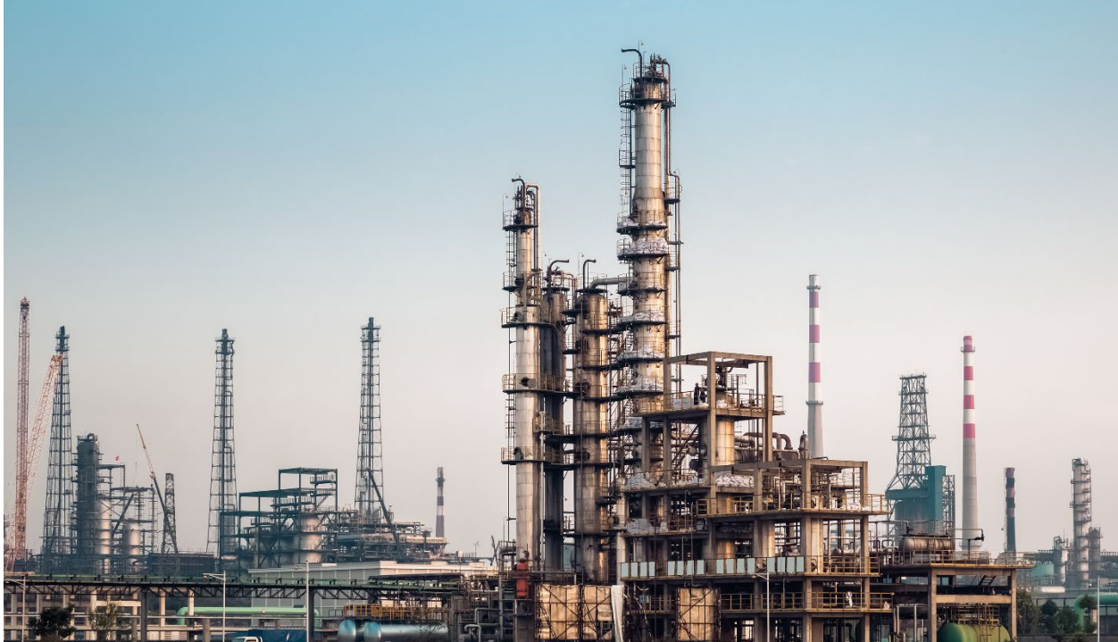
Figure 25: Industrial chemical plants – potential sites of chemical incidents – are located throughout the U.S.
