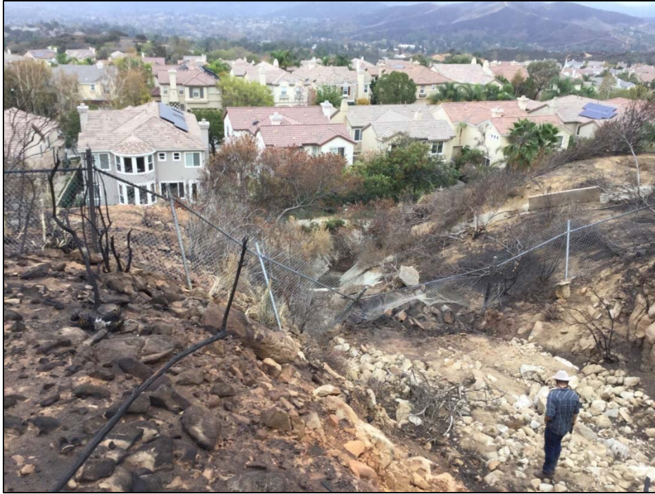
E-3. Oak Park existing hazard recorded by the WERT (Malibu Creek north region)
