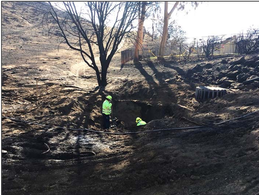
E-12. Wembly Avenue debris basin filled with sediment, Oak Park.
