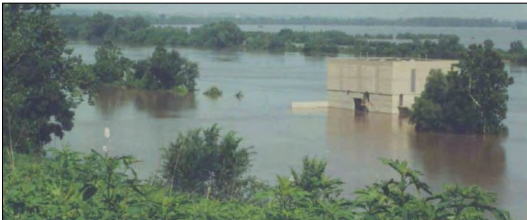
WaterOne's Isolated Intake during Floods in 1993.
