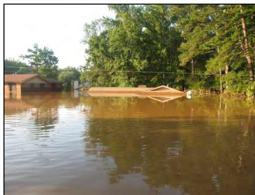
Flooded Houses on Windsor Drive in Douglas County, GA.
