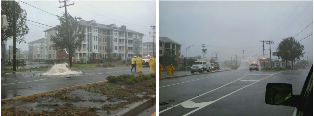
Water Main Break in Norfolk, VA During Hurricane Irene, 2011. Credit: City of Norfolk, Department of Utilities, 2011. Source: Tucker, 2014.
