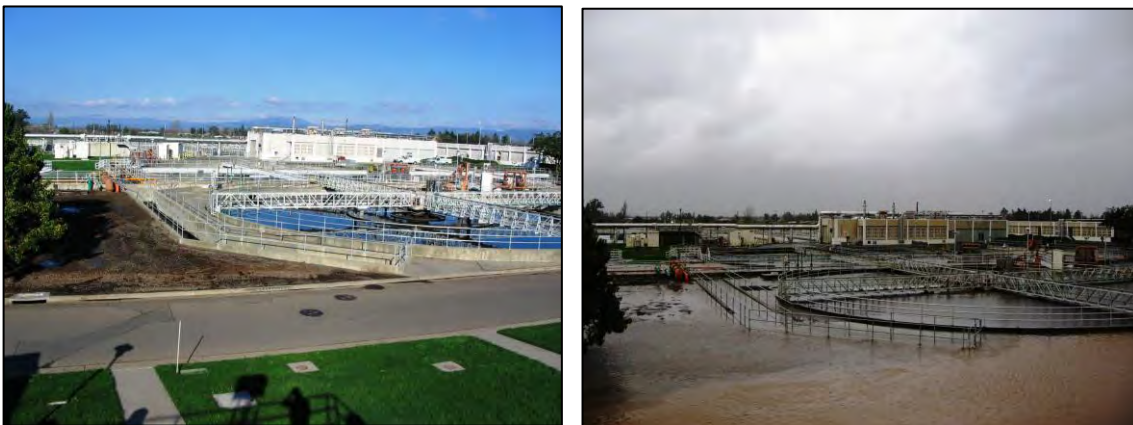
Santa Rosa Subregional Treatment Plant Normal Conditions (left) and during Flood 2006 (right).
