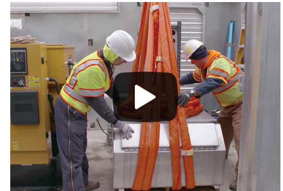
Video: Generator Placement
