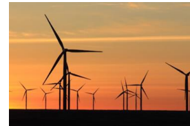
Figure 16. Traditional Wind Farm (courtesy of DOE)
