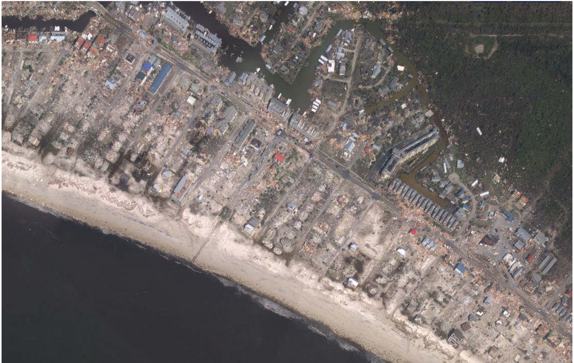
Figure 10. Aerial image of the devastation caused by Michael in Mexico Beach, Florida. Image courtesy of the NOAA National Geodetic Survey and the NWS Weather Forecast Office in Tallahassee, Florida.
