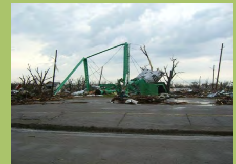
Photo: May 2007 Greensburg Tornado
